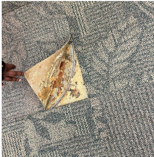
Cascades Photograph 6 – Location of a Slab Opening
