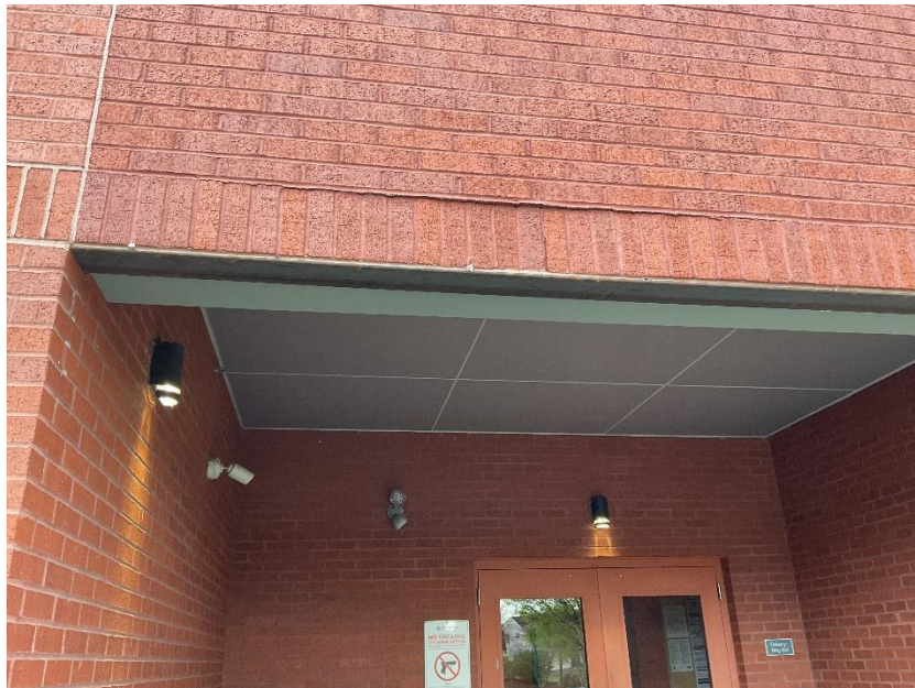
Ashburn Photograph 4 – Lintel above Loading Dock
