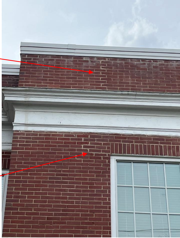
Administration Photograph 3 – Brick Repair
