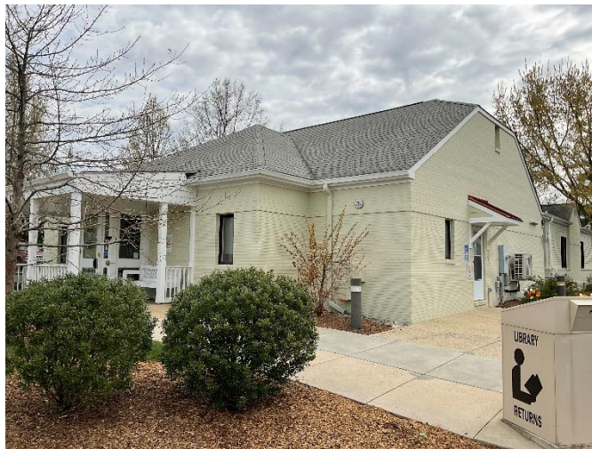
Lovettsville Photograph 2 – Building Exterior / Roof (SE Corner)
