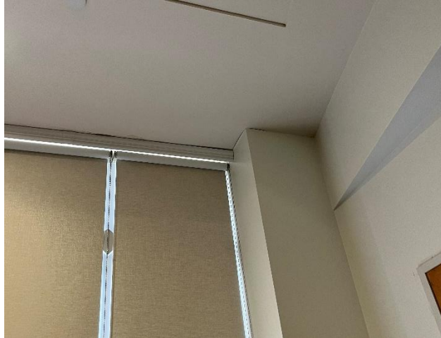
Cascades Photograph 3 – Separating Interior Finishes Near Door
