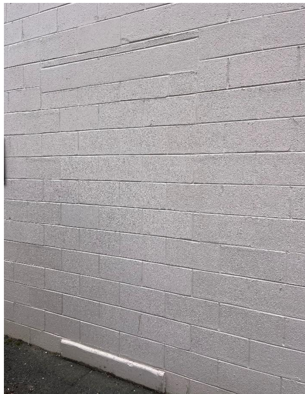
Sterling Photograph 2 – Masonry Infill at Opening
