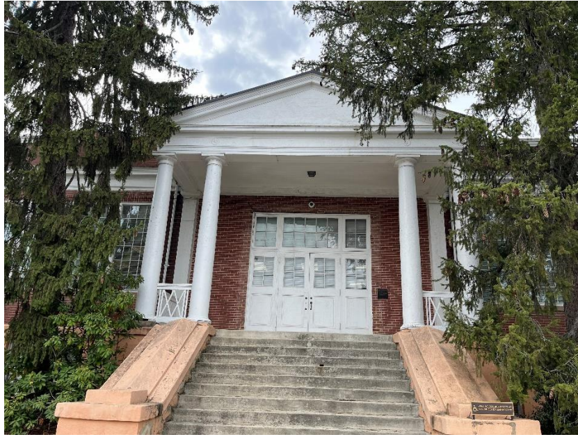
Administration Photograph 1 – Stair, Porch, and Porch Roof
